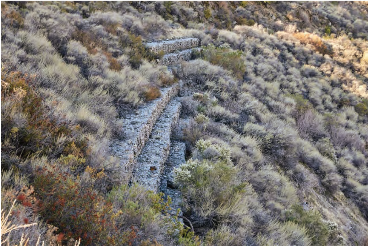
Figure 4-27. Gabion Retaining Walls
