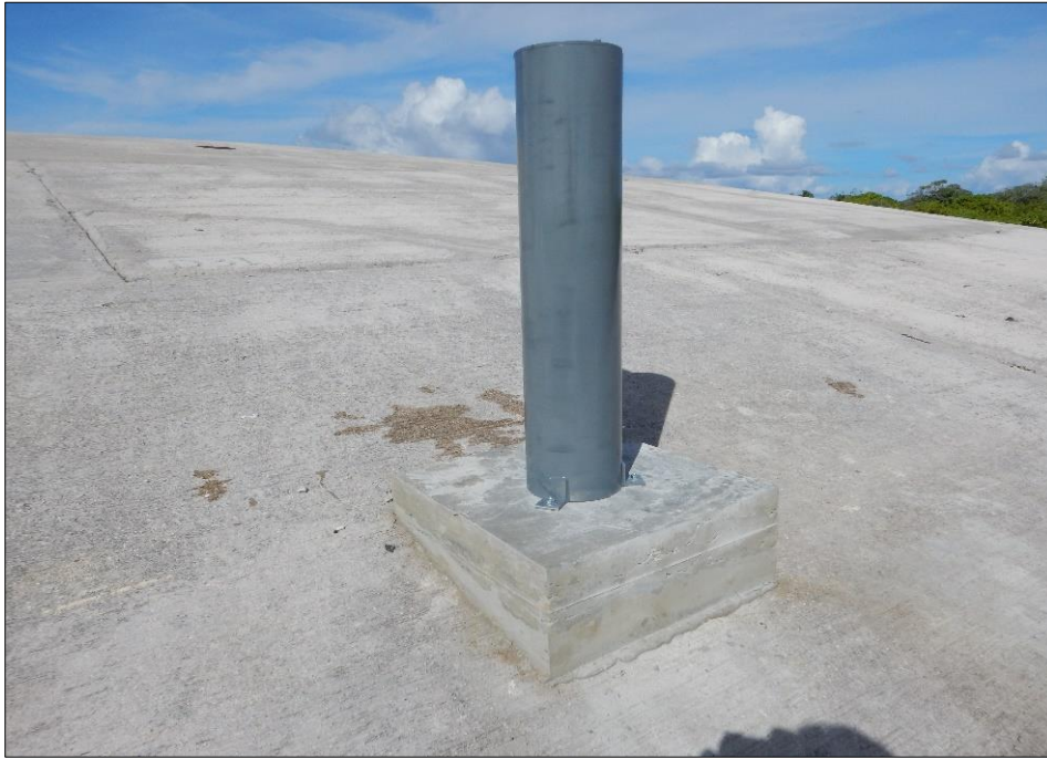
Fig. 1. Reconstituted CD-17 NAS Borehole on the Cactus Crater Containment Structure (after NAS, 1980)
