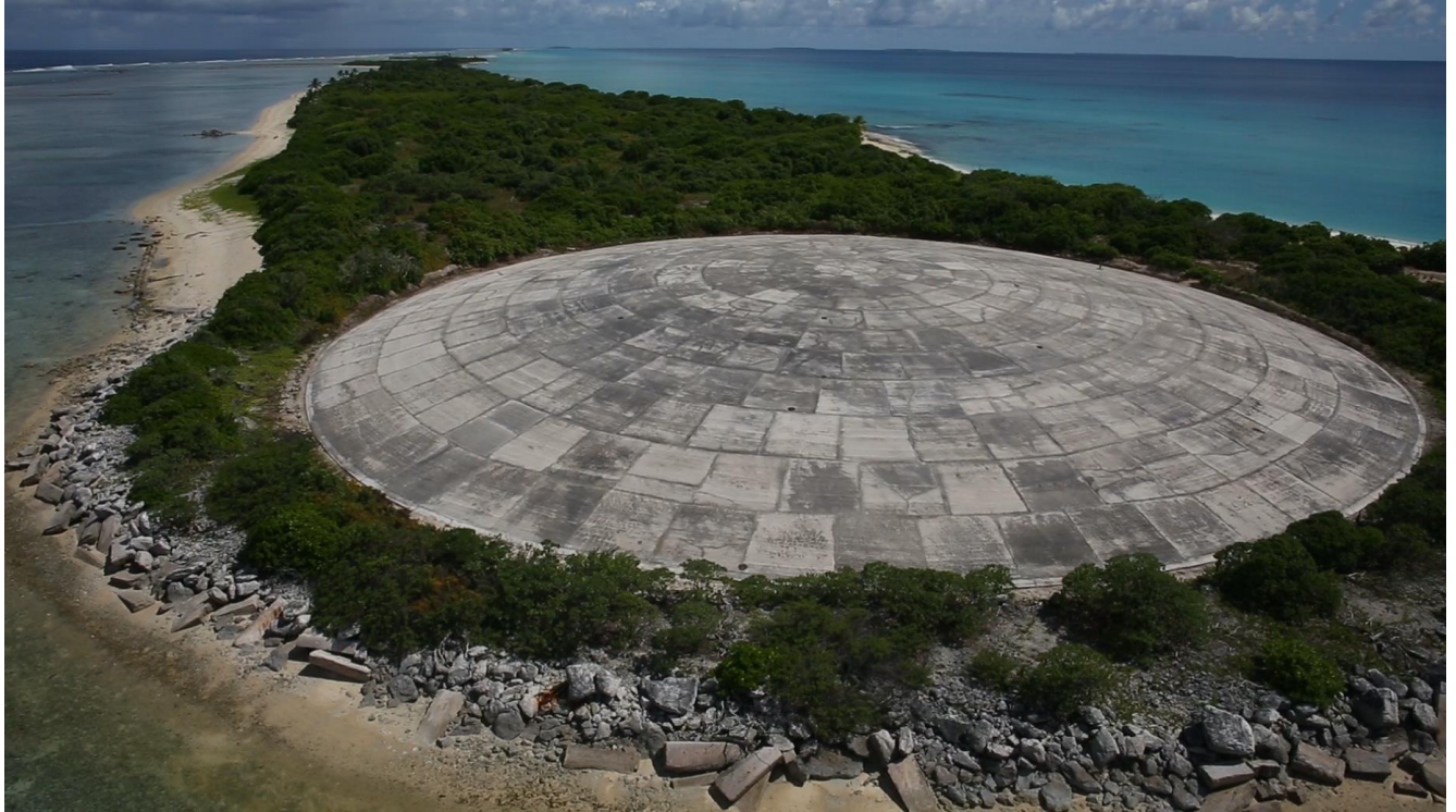
UAS Photo of the Cactus Crater Containment Structure (October 2018)
