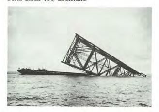
FIGURE **75.** Tilt-up Platform in Process of Being Erected
