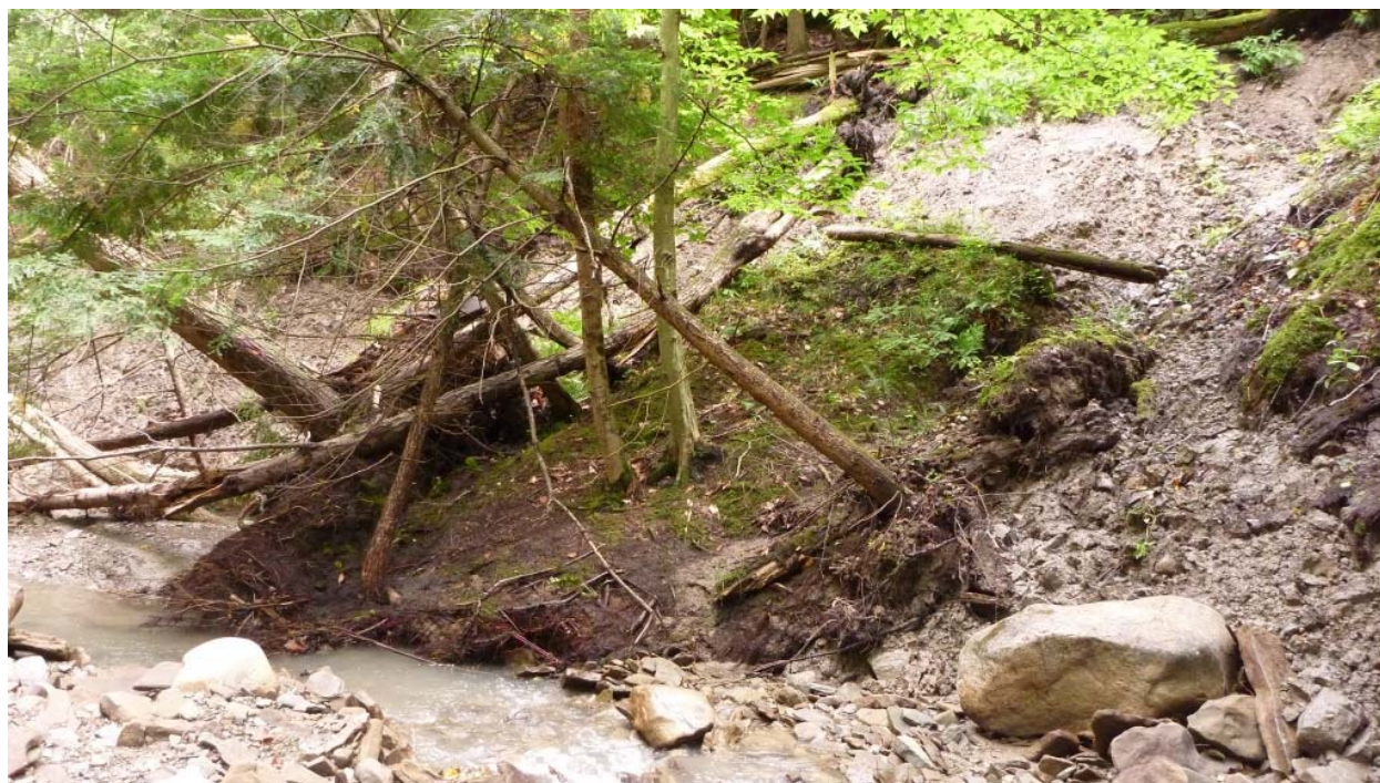
Figure 28. Abrupt slope failure as trees and root-bound soil slide down stream bank destabilized by erosion during 2009 flood. (Photograph courtesy of NYSERDA.)
