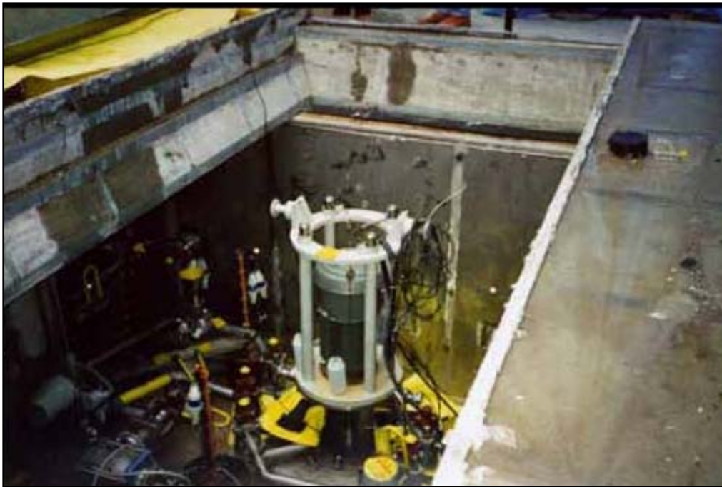
Figure 3-34. Typical HLW Pump Pit
