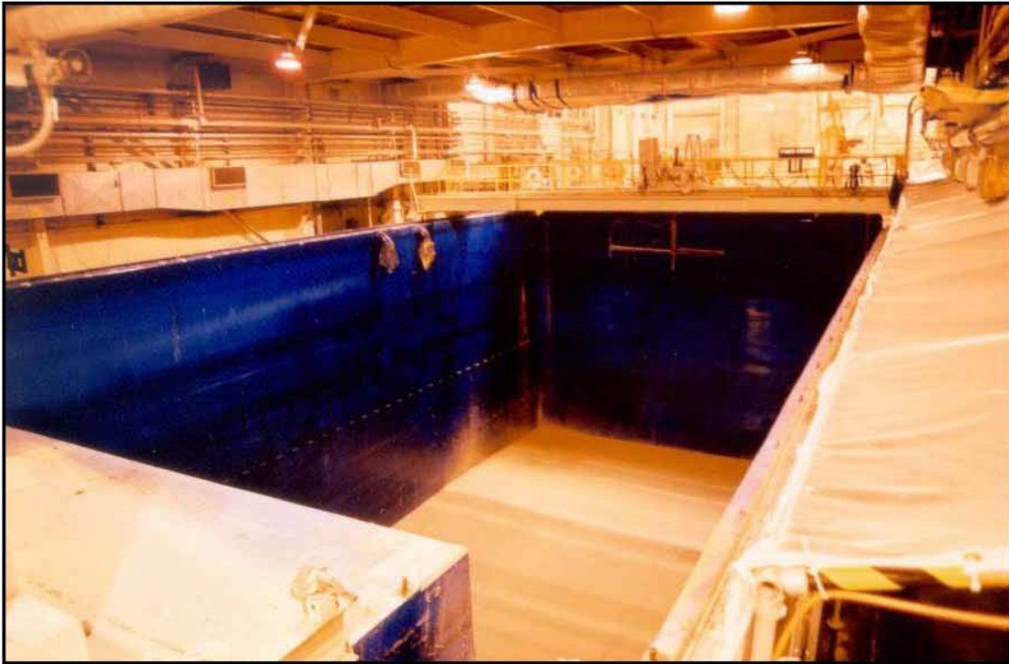
Figure 3-20. The Spent Fuel Pool After Deactivation
