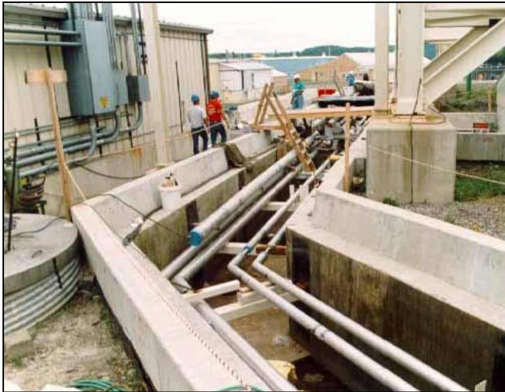
Figure 3-33. HLW Transfer Trench Under Construction
