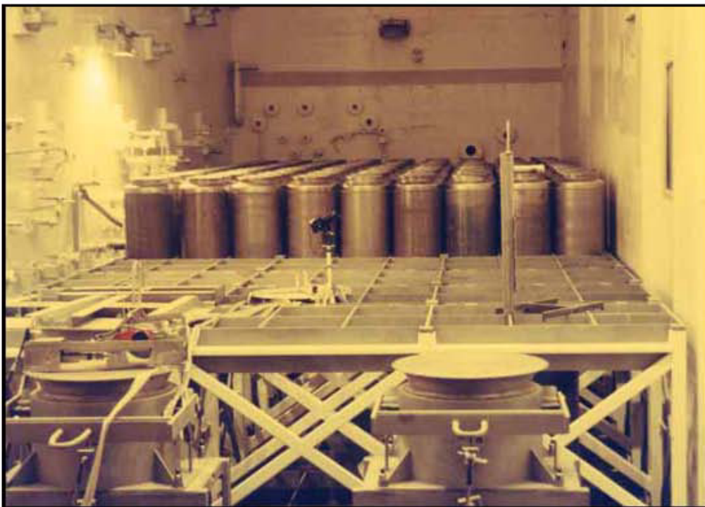
Figure 3-16. HLW Canisters Stored in the HLW Interim Storage Area
