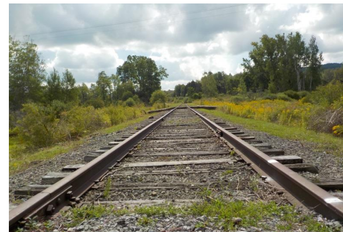
Vegetation Cleared on Rail Spur
