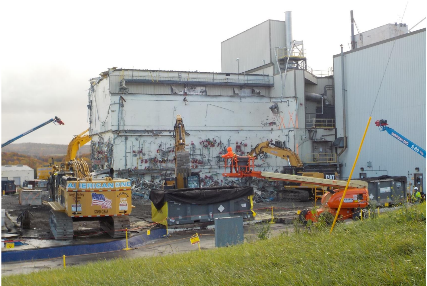
Vitrification Facility West Side – October 24, 2017
