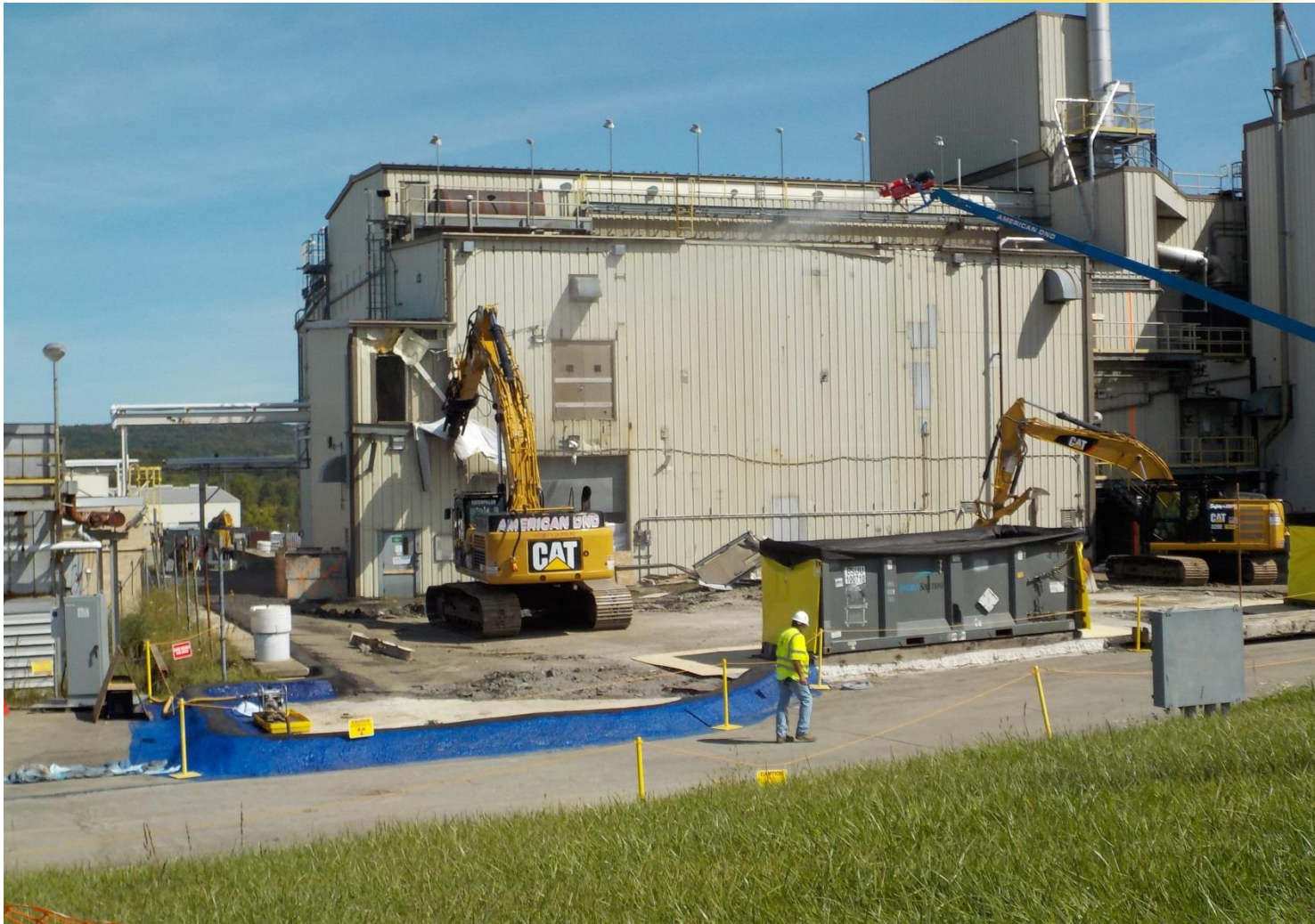
Vitrification Facility Demolition Start – September 11, 2017
