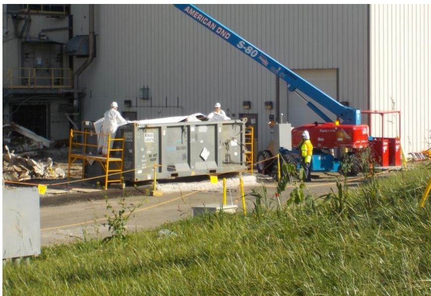
Vitrification Facility Waste Box Closure at the Demolition Site
