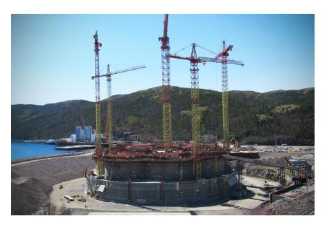
Figure 6: Construction of the Hebron concrete GBS at the Bull Arm site, Newfoundland (Photo: ExxonMobil Canada)
