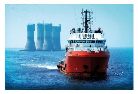
Figure 5: Towing of one of the Sakhalin II concrete GBSs from Vosthosny Port to field location outside Sakhalin Island (Photo: Sakhalin 2)
