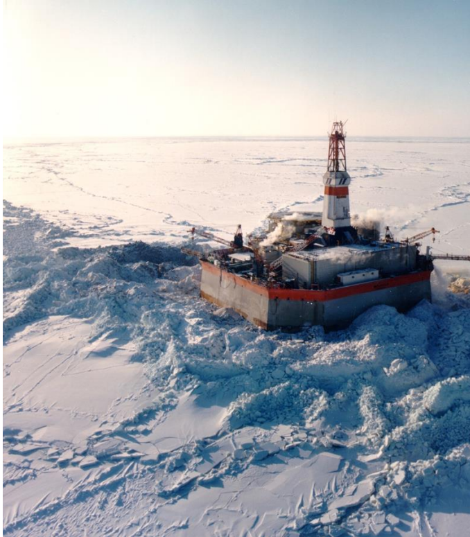
Figure 8. Example ice rubble field around the Molikpaq platform. (Photo: Canmar via Beaudril)
