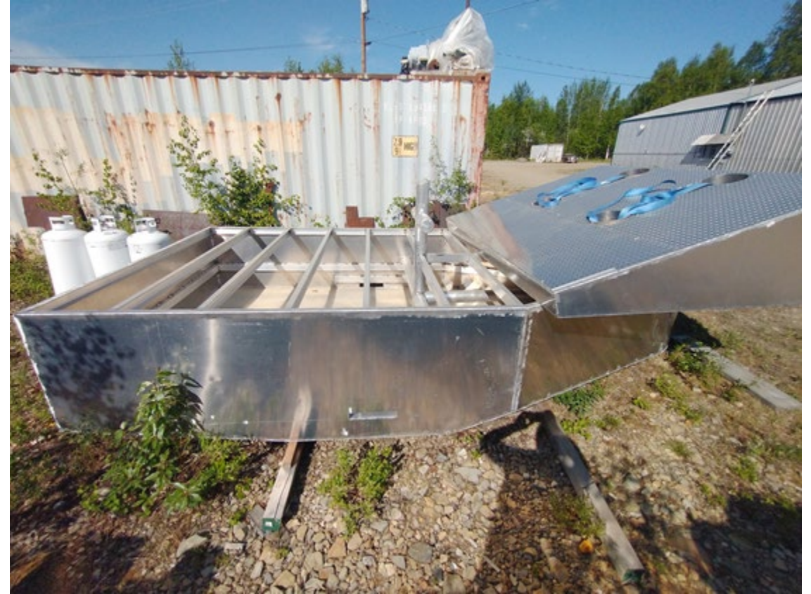
New debris diverter under construction
