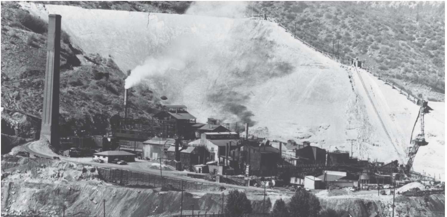
Durango mill during active operations (date unknown). The smokestack for the old lead smelter is to the left, with the large tailings pile and conveyances across the center.
