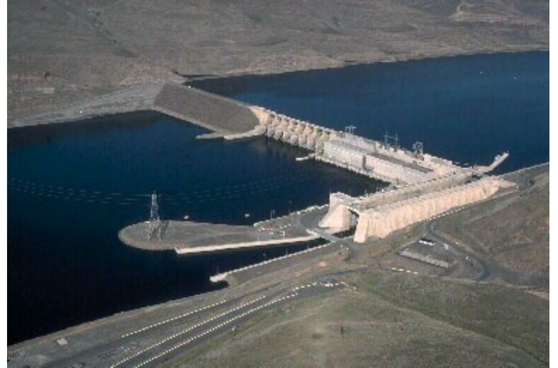
Little Goose Dam on Snake River in Lacrosse, WA
