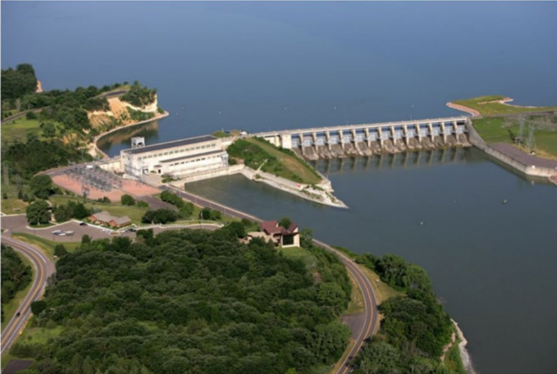
Figure 1. Aerial view of Gavins Point dam and power-house (source: Omaha District Hydropower Master Plan August 2016)
