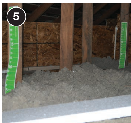
Insulation depth rulers installed, 1 per 300 square feet.
