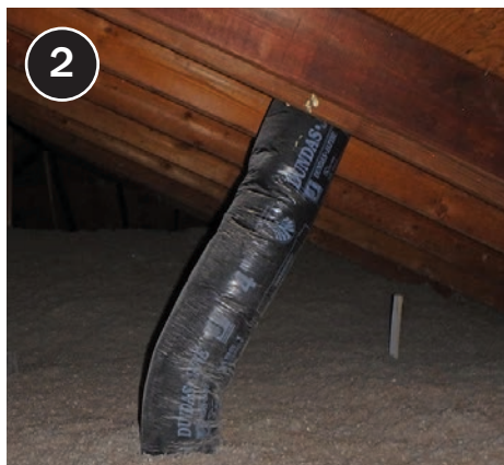
Route exhaust fan ducts to outside, insulate the ducting to R-8.
