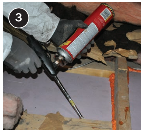
Ensure air sealing work is complete prior to adding insulation.
