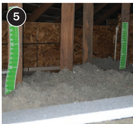
Insulation depth rulers installed, 1 per 300 square feet.
