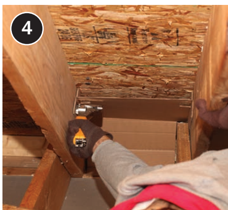
Install baffles, if needed. Ensure 1–2 inches of space between the baffle and roof decking for airflow.
