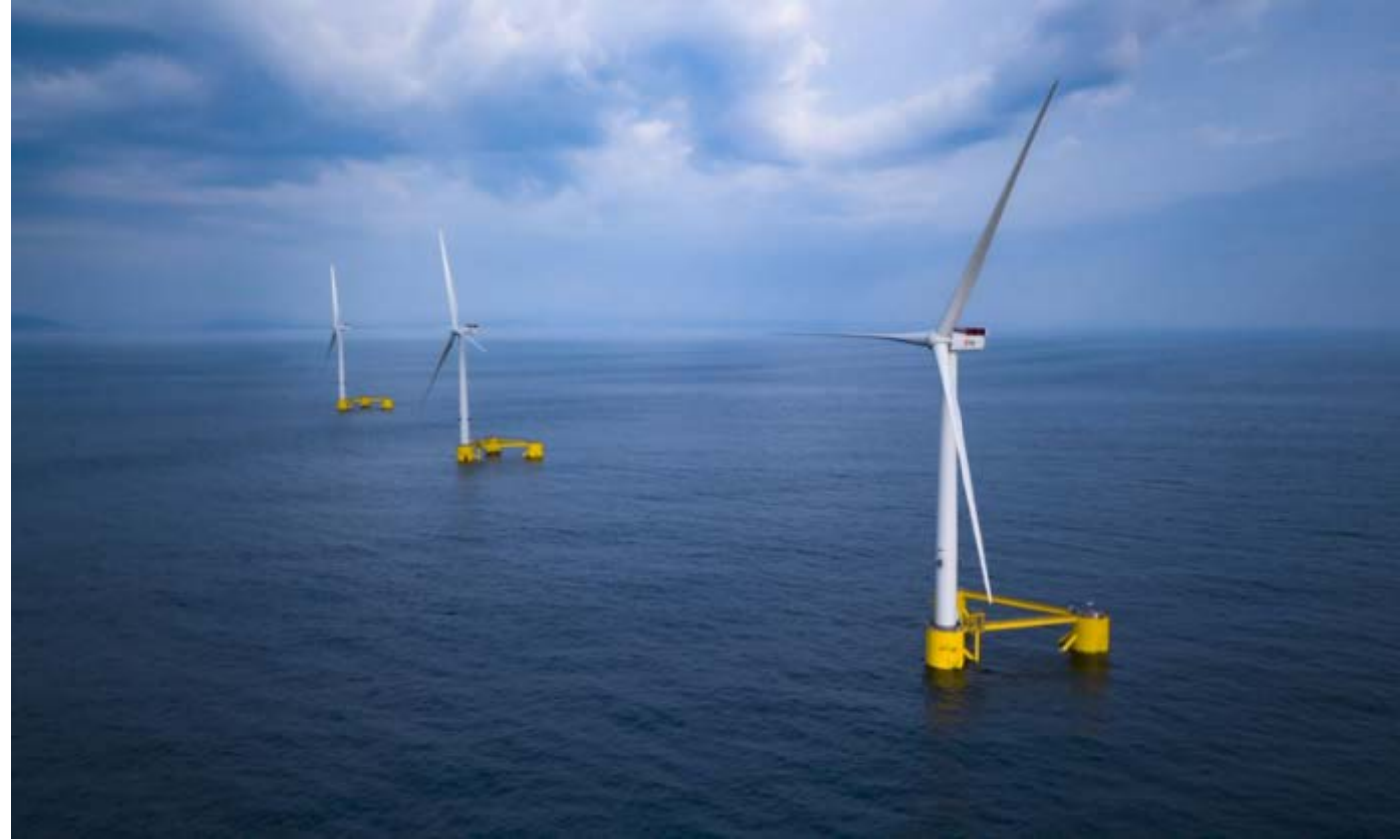
Kincardine 47.5-MW Floating Offshore Wind Plant
