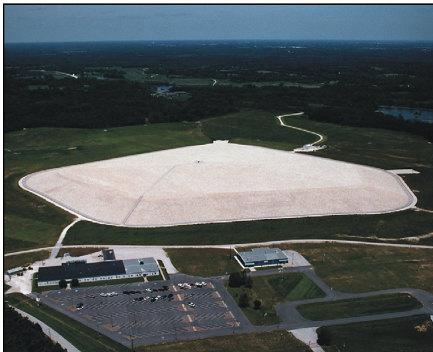
Weldon Spring Disposal Cell circa 2002.
