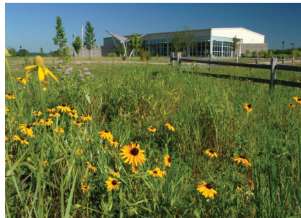
Fernald Preserve Visitors Center, Ohio
