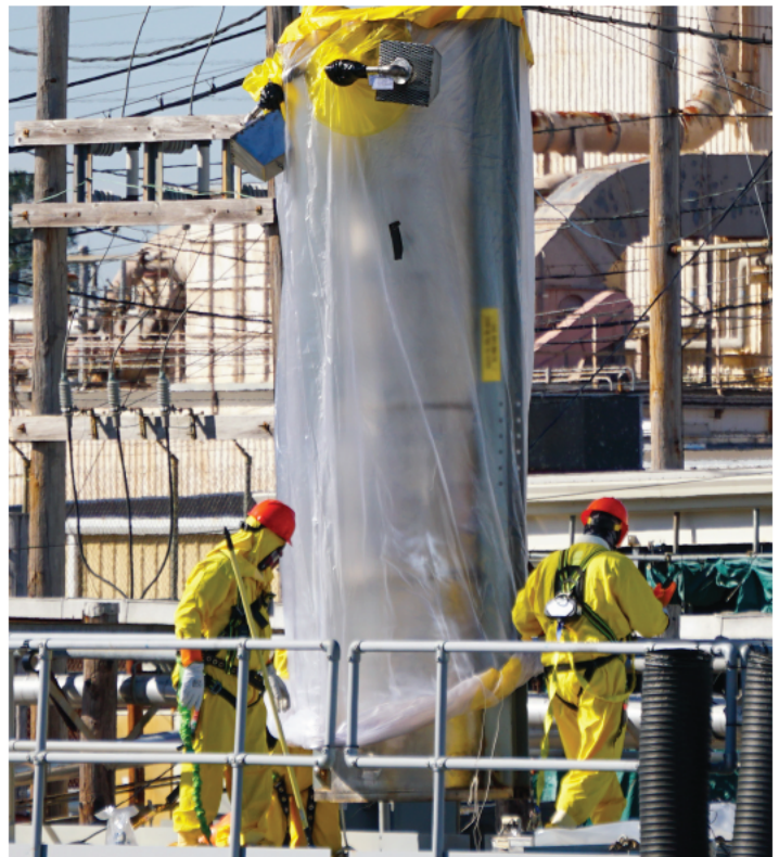
TCCR utilizes ion-exchange columns to remove cesium from liquid waste.
