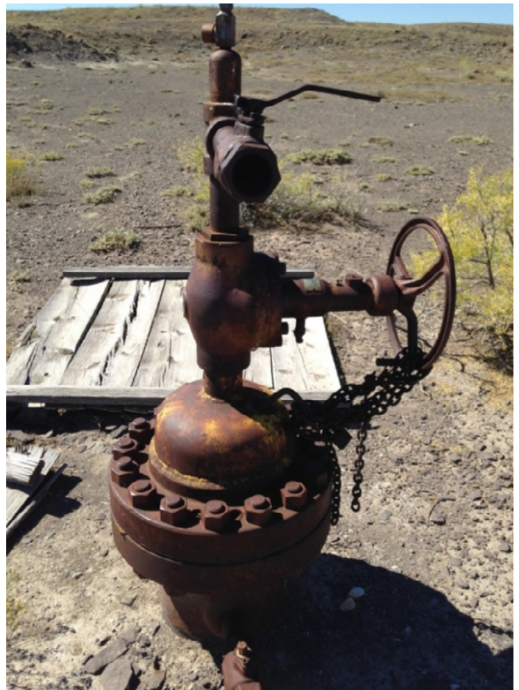
Utah, Utah, Site Wellhead, Looking South, September 27, 2016.
