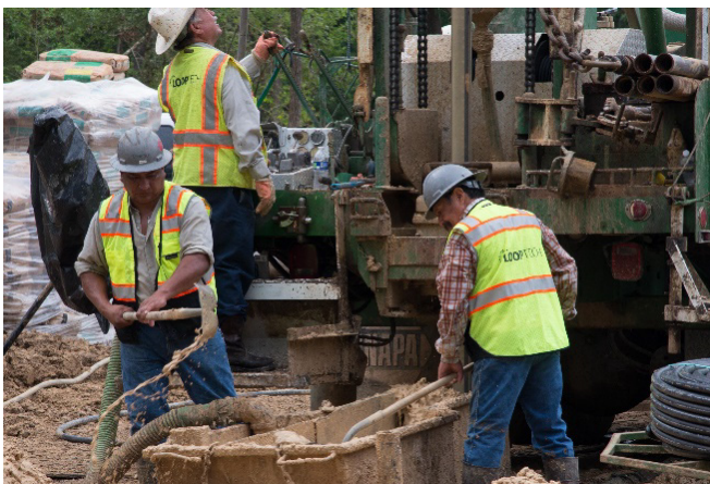
Figure 7. HARC's GSHPs use Houston's near-constant, below-ground temperature of about 72°F (Olgun 2015) to dispel or absorb heat. Photo: HARC
