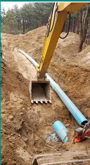
Photo: Installation of underground piping connecting groundwater extraction wells to a PFAS treatment system at BNL.
