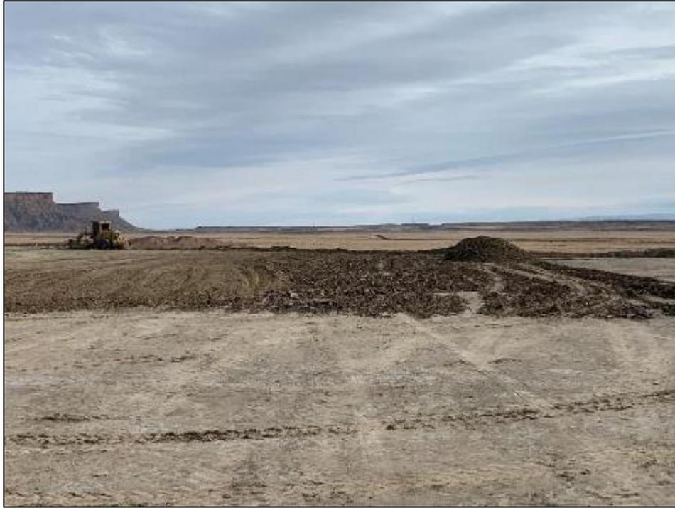
*Photo 33. Placing Protective Cover on Interim Cover November 2019*
