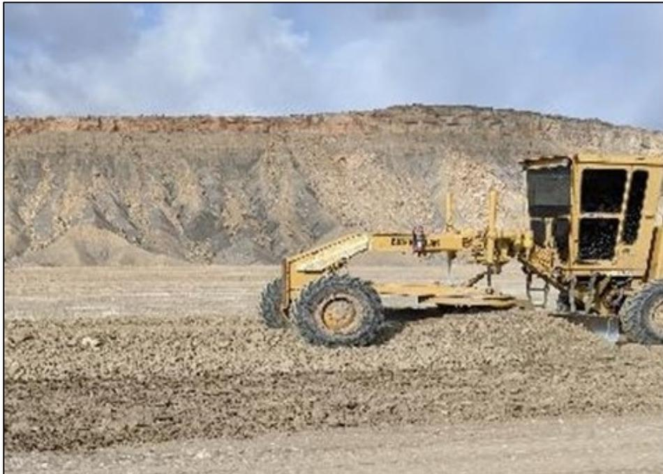
*Photo 34. Grader Placing Protective Cover on Top of Interim Cover December 2019*
