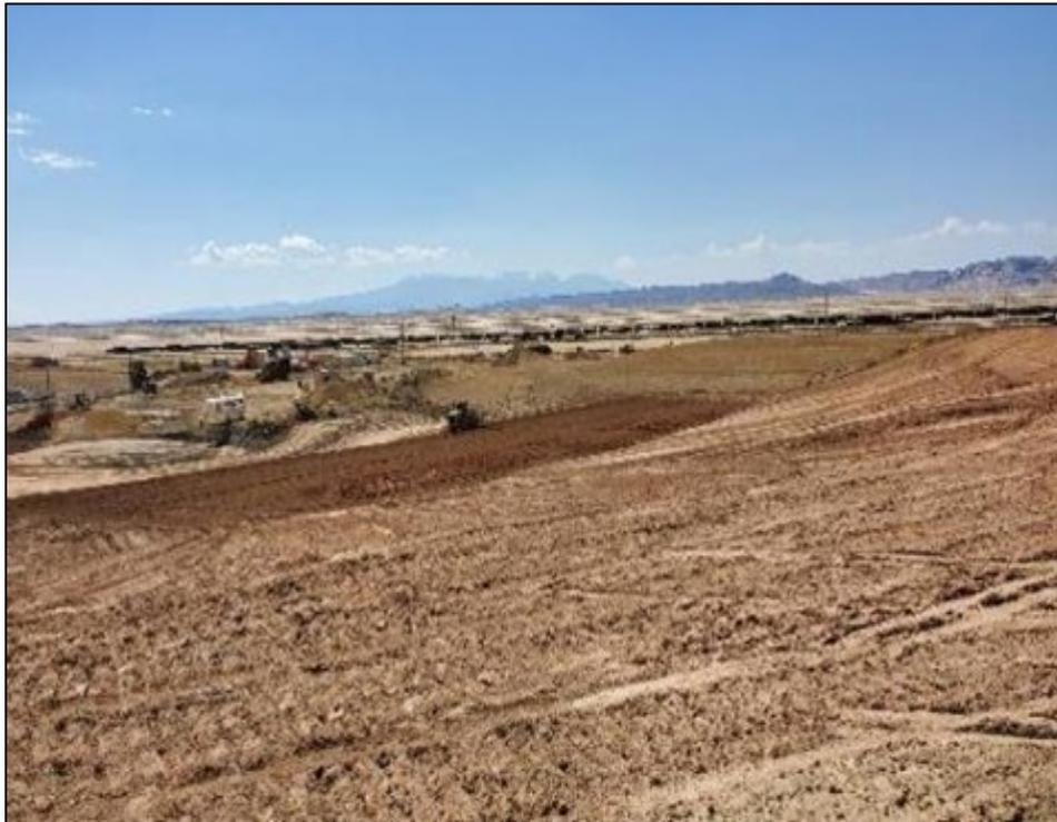
*Photo 22. Compacting Lift Area with Sheepsfoot June 2020*
