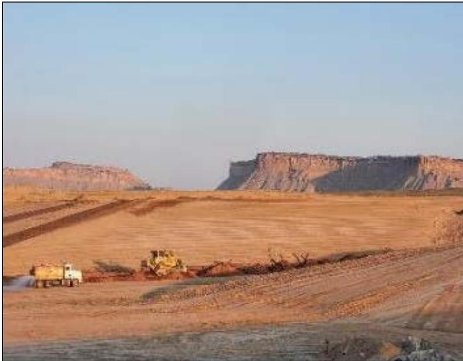
*Photo 28. Bulldozer Placing Material for 2 Foot Debris Lift August 2020*
