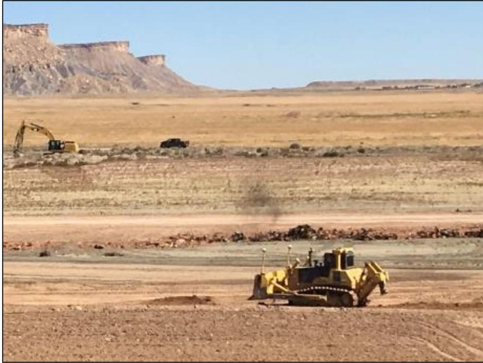
*Photo 5. Bulldozer Pushing Material To Be Compacted October 2019*
