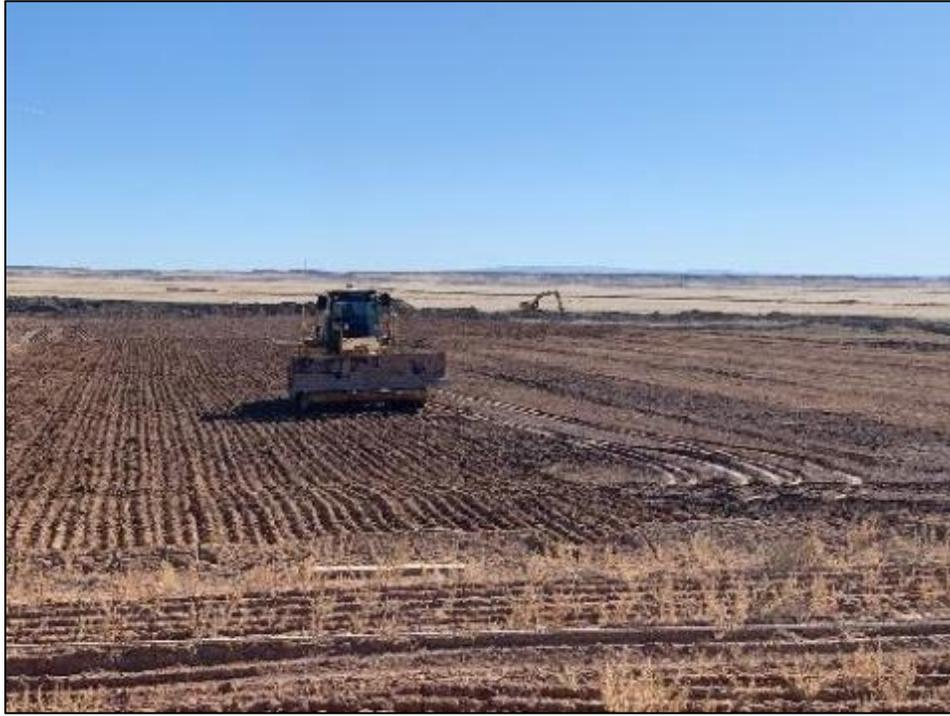
*Photo 14. Compacting North Top of Seven Foot Lift March 2020*
