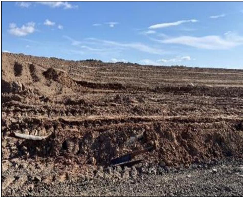
*Photo 12. Two Foot Sacrificial Lifts on Floor of Cell    January 2019*
