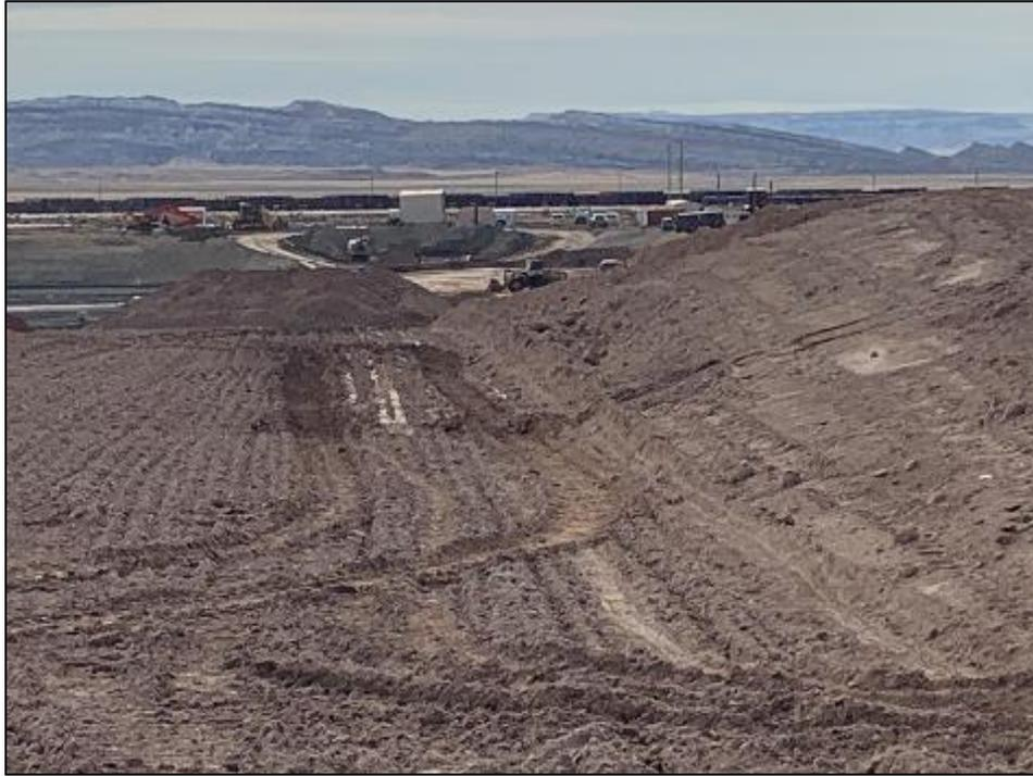
*Photo 7 RRM Lifts Scarified for Prior to Placement November 2019*
