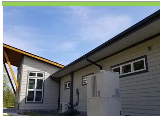
The Eklutna Village Medical Clinic's 5 kW Yanmar reciprocating engine-based CHP system Photo from Eklutna Village Medical Clinic
