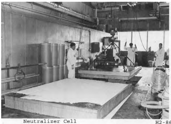
Figure 8-36. Photo H2-86, Removing Neutralizer Cell Access Hatch at the 332-Foot Level, undated
