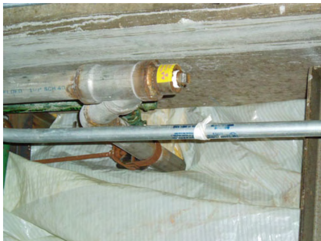
Figure 9-8. Photo TNL-10a, G1 Tunnel Capped Drain Pipe, 2004
