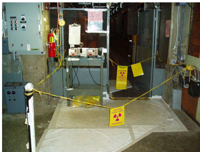
Figure 9-4. Photo TNL-8, E1 Tunnel Aisle Entry, 2004
