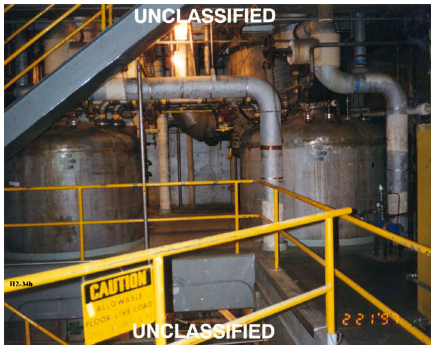
Figure 8-26. Photo H2-34b, 319-Foot Level East and West Receiver Tanks, undated
