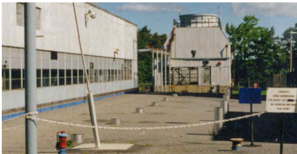
Figure 10-1. Photo H2-93, Tank Farm Area East of Building H2, Looking North, 2004
