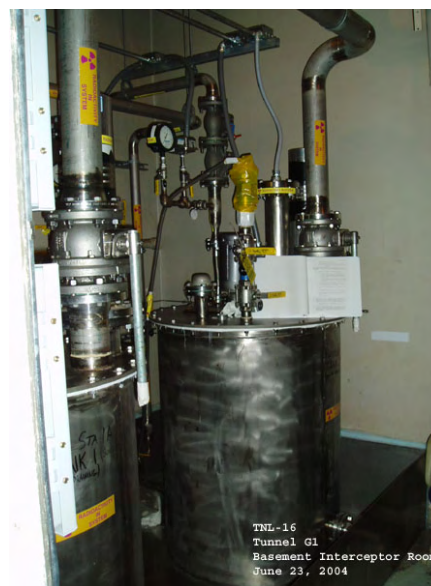
Figure 9-10. Photo TNL-16, New Interceptor Placed in G1 Tunnel, 2004
