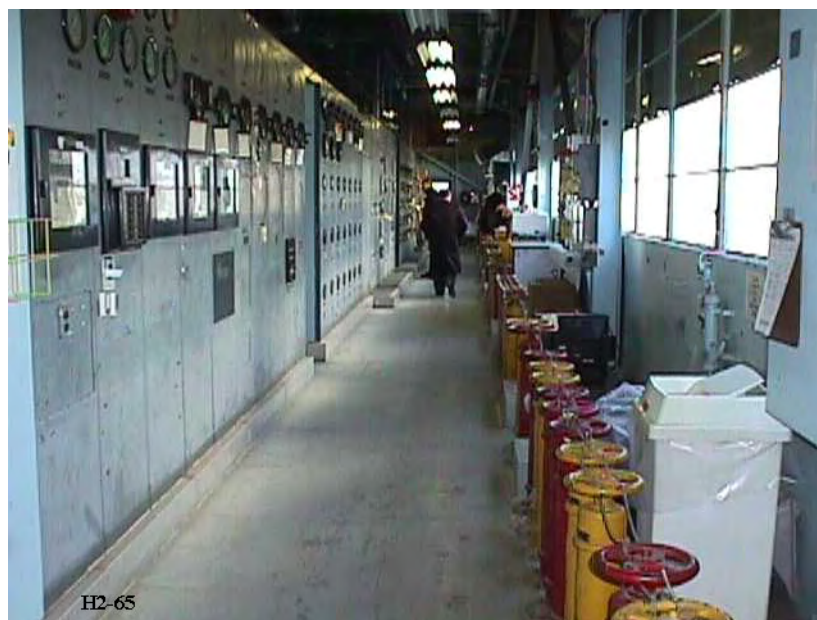
Figure 8-31. Photo H2-65, H2 Control Room and Entryway, 332-Foot Level, undated
