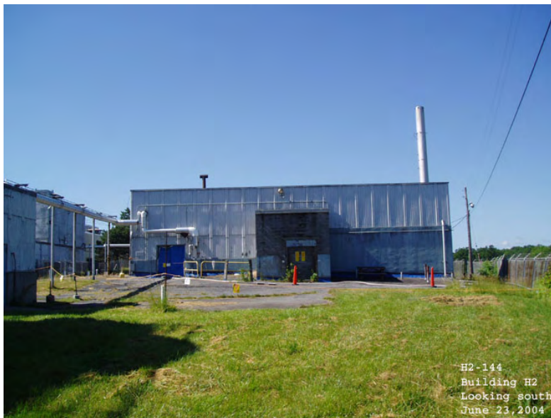
Figure 8-39. Photo H2-144, Slurry Drum Facility, North Side of H2, June 23, 2004
