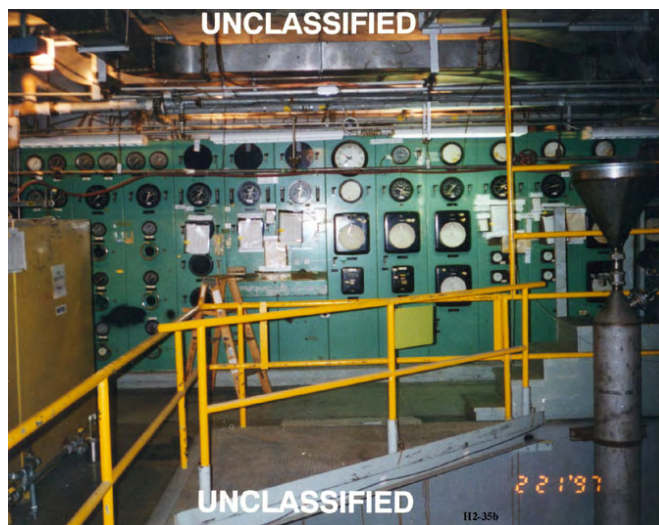
Figure 8-22. Photo H2-35b, 319-Foot Level Instrument Panel, undated
