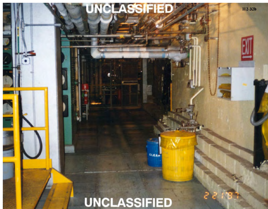
Figure 8-17. Photo H2-32b, Outside East Wall of the Former Drum Dryer Cell looking south, 319-Foot Level, undated
