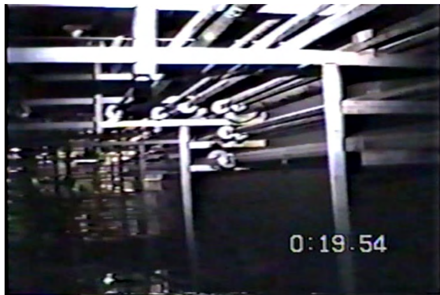
Figure 9-13. G2-H2 Tunnel Structure and Piping, July 1989 (V-002008)
