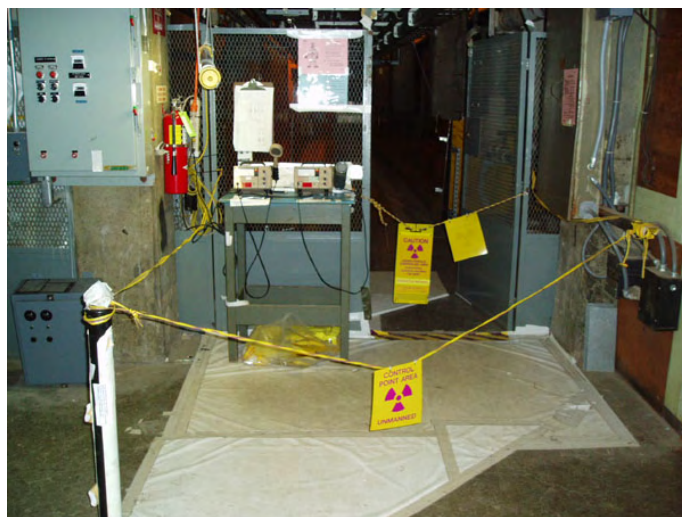
Figure 9-4. Photo TNL-8, E1 Tunnel Aisle Entry, 2004
