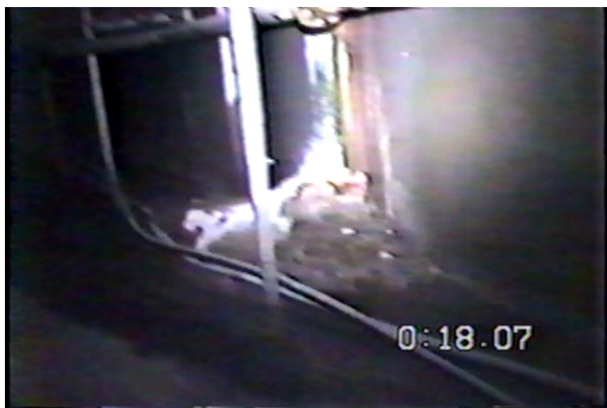
Figure 9-14. G2-H2 Tunnel Debris Pile, July 1989 (V-002008)
