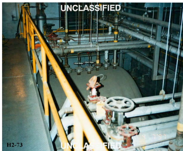
Figure 8-20. Photo H2-73, Evaporator Storage Tank Area, 319-Foot Level Looking South, 1997
