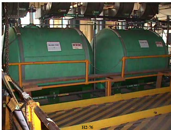
Figure 8-35. Photo H2-76, Hillside Drain System Tanks and Neutralizer Hatch, undated
