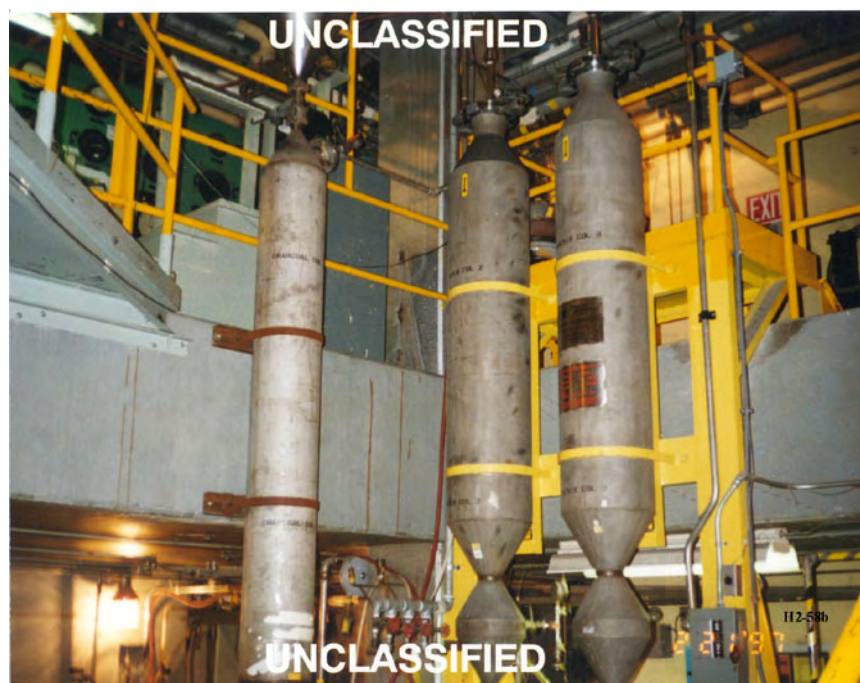
Figure 8-27. Photo H2-58b, Radioactive Materials Laboratory Reuse System Ion Exchange Tanks, 309- and 319-Foot Levels, undated
