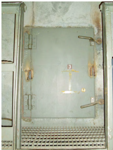
Figure 9-7. Photo TNL-11, G1 Tunnel Welded Hatch, 2004
