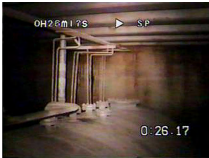
Figure 10-4. Tank Top in Tank Farm Vault, Looking East, undated
