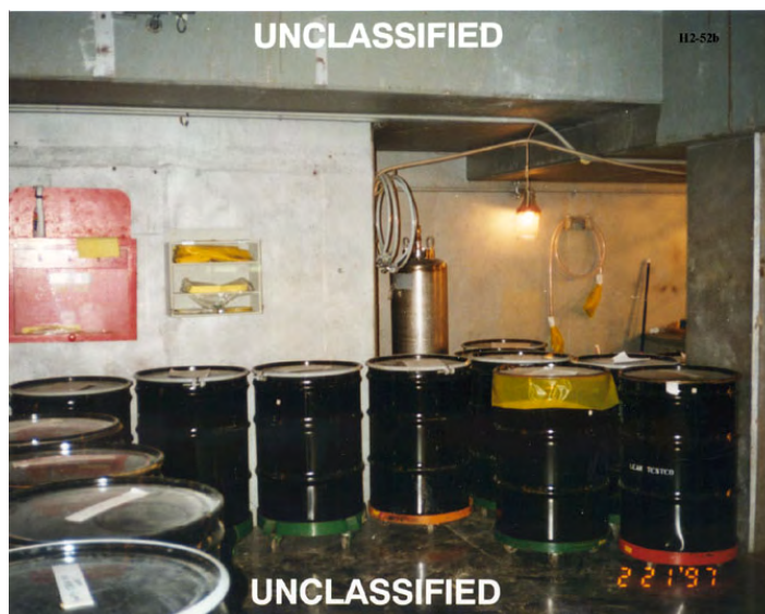
Figure 8-41. Photo H2-52b, 309-Foot Level Viewing the North Door and Waste Drums, undated
