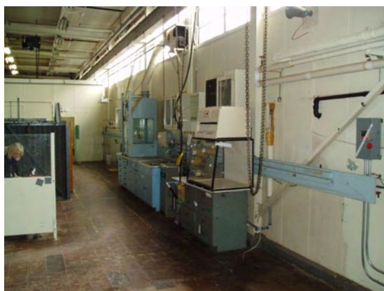
Figure 7-73. Photo G2-158, G2 357-Foot Level, Crane Gallery, West Wall, November 2004
