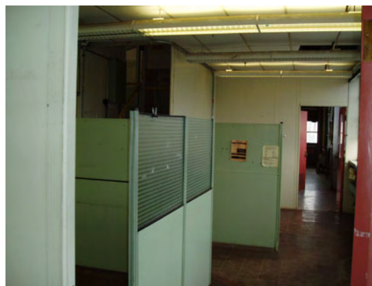
Figure 7-72. Photo G2-153, G2 357-Foot Level, Room 199 South End, November 2004
