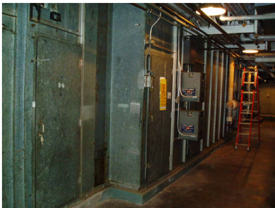
Figure 7-80. Photo G2-162, G2 357-Foot Level Ventilation Room, Looking West, November 2004
