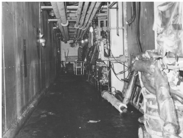
Figure 7-39. Photo G2-59, Lower Sample Aisle – Looking South (KS-60544), Post-SPRU Decommissioning, undated
