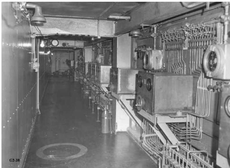
Figure 7-65. Photo G2-38, G2 348-Foot Level, Upper Sample Aisle Looking South, undated
