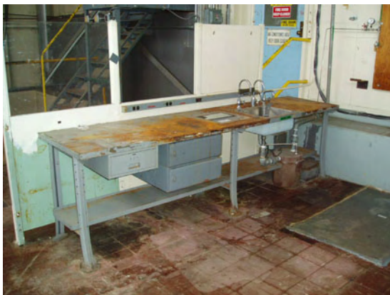
Figure 7-75. Photo G2-155, G2 357-Foot Level, Crane Gallery, East Wall, November 2004
