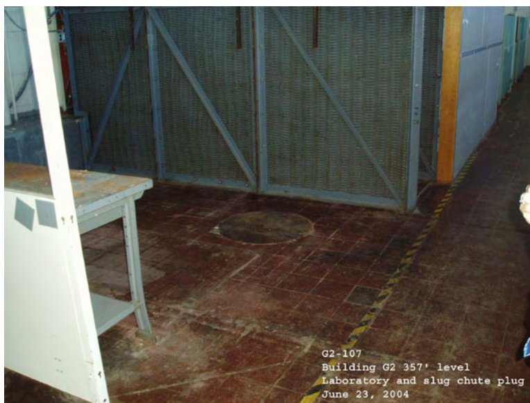
Figure 7-85. Photo G2-107, G2 357-Foot Level Laboratory and Slug Chute Plug, June 2004
