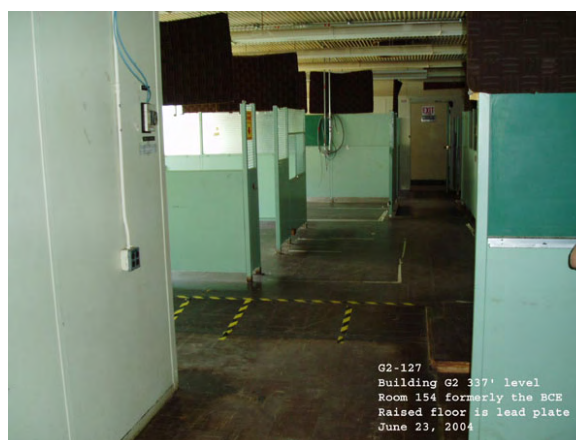
Figure 7-48. Photo G2-127, G2 337-Foot Level, Room 154 formerly the BCE, June 2004
