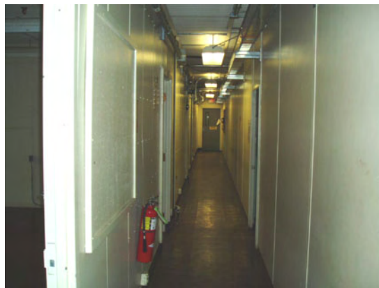
Figure 7-88. Photo G2-154, G2 357-Foot Level, Corridor, November 2004
