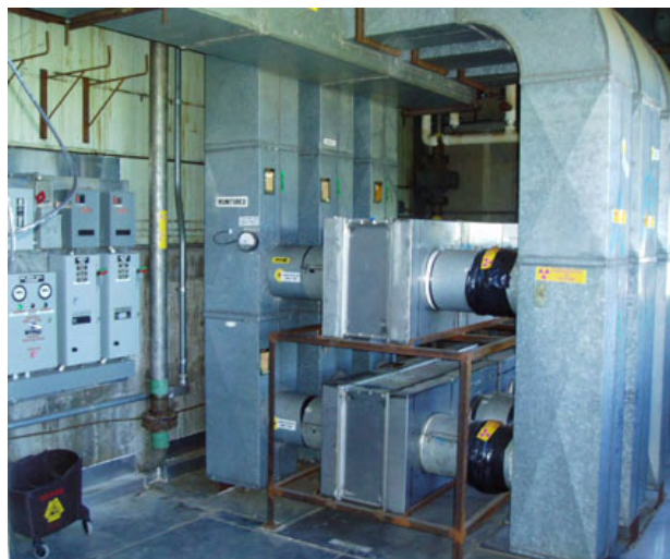
Figure 7-78. Photo G2-105, G2 357-foot Level, Equipment Room, November 2004
