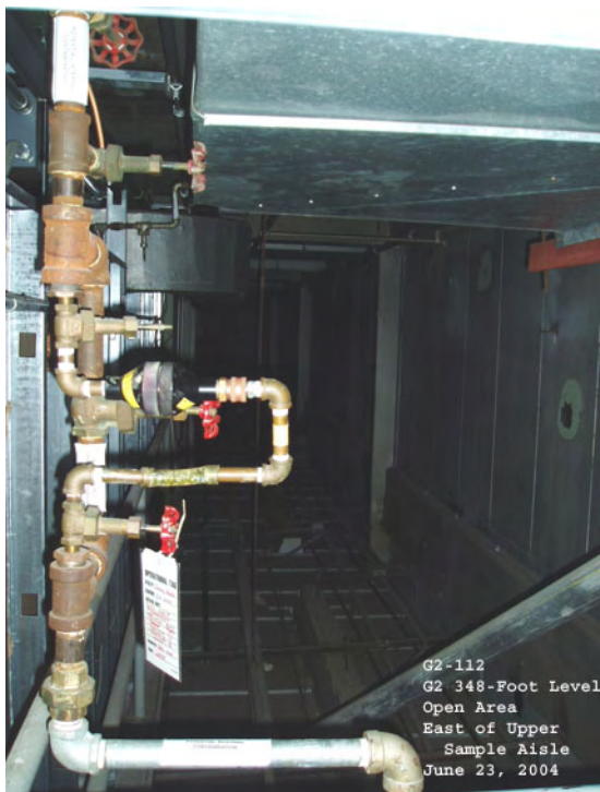
Figure 7-61. Photo G2-112, G2 348-Foot Level Open Area East of Upper Sample Aisle, undated
