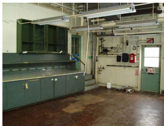
Figure 7-74. Photo G2-157, G2 357-Foot Level, South End of Crane Gallery, November 2004
