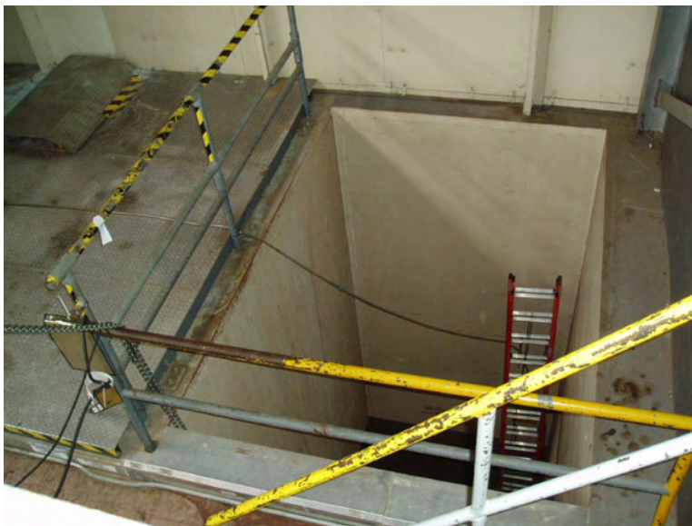
Figure 7-37. Photo G2-164, G2 Overlooking Hoisting Bay from 357-Foot Level, November 2004
