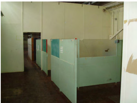
Figure 7-87. Photo G2-159, G2 357-Foot Level, Office Space Center-West, November 2004
