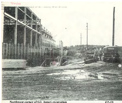
Figure 7-7. Photo G2-19, G2 Under Construction Shows Steel Framing and Concrete Walls, July 20, 1948
