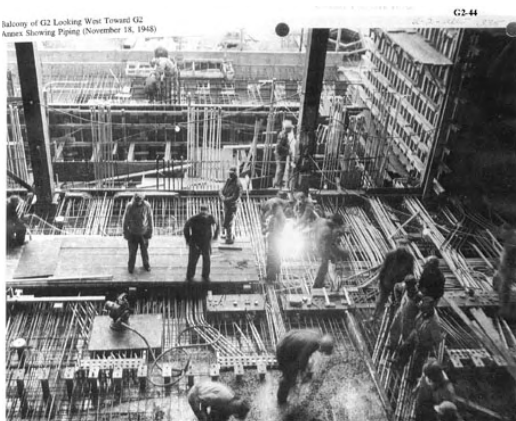
Figure 7-5. Photo G2-44, Balcony of G2 Looking West Toward G2 Annex Showing Piping, November 18, 1948
