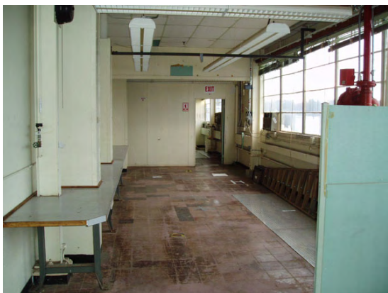
Figure 7-33. Photo G2-143, G2 337-Foot Level, Room 197 View 2, November 2004
