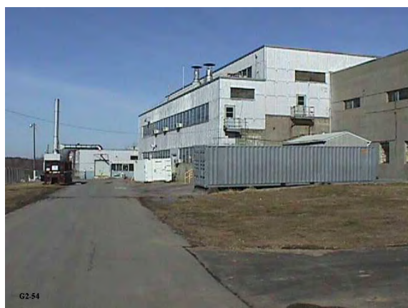
Figure 7-3. Photo G2-54, G2 South and West Sides (Looking North), November 2004
