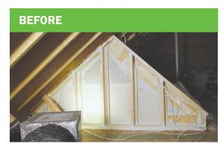
Install durable backing material into any large gaps before applying spray foam to prevent foam from leaking into conditioned space. All surfaces in contact with foam should be free of dust and debris. Ventilate the work space according to manufacturer specifications to ensure workers and occupants are protected from spray foam vapors during and after installation.
