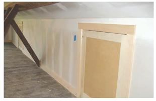
Separate all foam products from living space with a thermal barrier material such as 1/2 inch drywall. Additionally, if the attic is only used for the service of utilities, foam will be separated from the attic space using a suitable ignition barrier. If the attic space is used for storage or occupancy, spray foam will be separated from the attic using a suitable thermal barrier.
