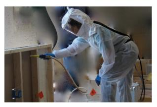
Ensure installers are wearing appropriate personal protective equipment (respiratory, skin/body, and eye). Follow the manufacturer's specified temperature guidance for ambient air, surface, and chemical to avoid product failure.
