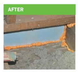
Air sealing each and every open joist cavity below the knee wall prevents air movement between the unconditioned attic and the conditioned floor.
