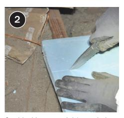
Cut blocking material (extruded polystyrene, wood, gypsum board) to fit gap.
