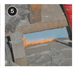
Seal around the edges of the blocking material to align the pressure boundary.
