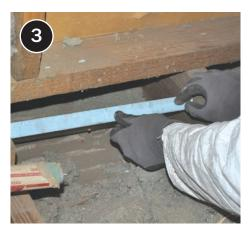
Securely fit infill or blocking material in place.
