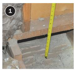
After clearing away debris, measure gap below knee wall in line with pressure boundary.
