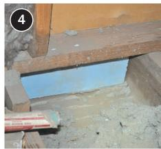
Ensure blocking material is located in line with preferred pressure boundary.
