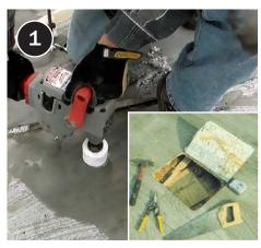
Cut access holes (rectangular or round holes) large enough to fit a fill tube in each cavity.
