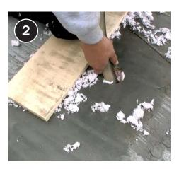
Carefully insert a fill tube or pipe and insulate all areas to the correct density using fiberglass insulation.
