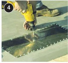
Install a bead of sealant and mechanically fasten a metal patch in place.
