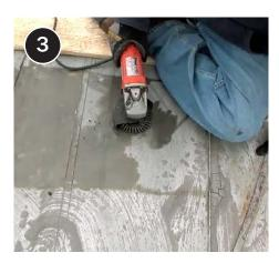
Prepare the area around the hole before installing a metal patch.
