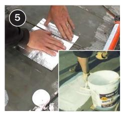
Install a flexible adhesive roof patch over the first patch. When complete, apply a final coat of elastomeric paint over the affected area.
