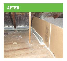
An insulated attic floor provides a continuous, contiguous, safe, and compliant thermal boundary that reduces air movement.
