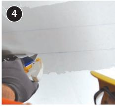
Occasionally, a homeowner may not want the attic floor to be disturbed. The cavities can also be accessed from below through the ceiling, particularly in garages.
