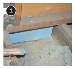
Ensure that floor cavities and chases are blocked securely at both ends with all edges of the blocking sealed.
