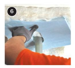
Blow insulation to completely fill cavities to prescribed density.
