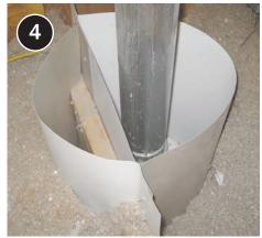
Ensure that insulation does not get into dammed-off areas, such as around chimneys and flues and inside soffit baffles.
