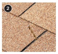
Locate the ideal location for the vent and, from the attic side of the roof, drill a small pilot hole centered between the roof rafters. Exterior exhaust terminations should be located at least 3 feet from property lines, operable openings (windows and doors) to the home, and at least 10 feet from mechanical intakes or distances specified by the authority having jurisdiction.
