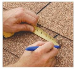
Mark out size and location of hole on roof deck, verifying size of termination collar.
