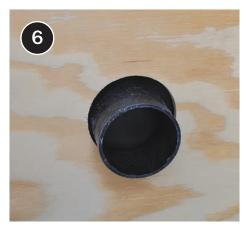
Collar should extend down through roof into attic.
