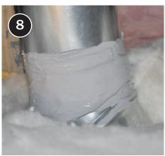
Seal duct joints with mesh and mastic to complete vent installation. Insulate as required.
