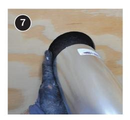
Slide vent ducting to collar, sized to match the duct diameter, and attach with mechanical fasteners.
