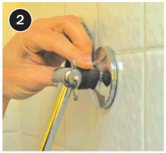
If old showerhead does not have flat sides at connection, wrap with buffer material, such as a piece of rubber.
