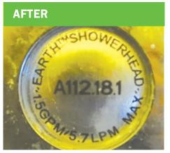
Low-flow showerheads must have flow rates of 2.5 gallons per minute or less, to reduce heating load and water use.
