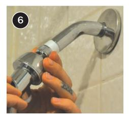
Install new showerhead according to occupant needs, such as handheld, shut-off, or swivel.
