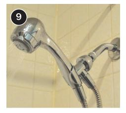
Verify proper water flow and that there are no leaks.
