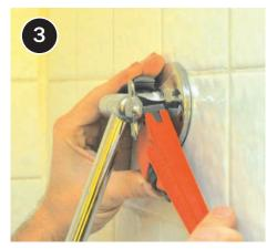
Then use pipe wrench or channel locks to loosen connection at shower arm.
