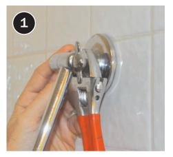
Carefully remove old showerhead with adjustable wrench, taking care not to loosen shower arm.
