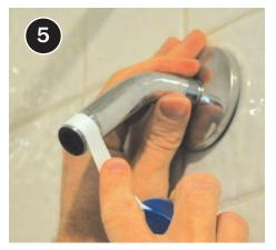
Wrap new thread tape around threads.
