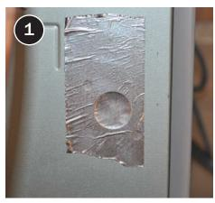
Cover any unnecessary holes in the air handler cabinet.
