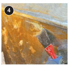
Prepare plenum by removing any residue from old insulation.
