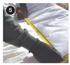
Measure insulation to take maximum advantage of large sheets of duct insulation.
