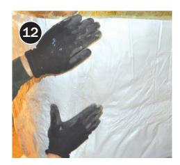
Ensure overlapping flap is securely attached to the lower layer to maintain a complete vapor barrier, or tape seams with UL-181 tape.
