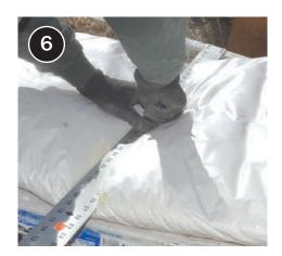
Cut to size for area to be covered. Insulate all exposed metal of the plenum.
