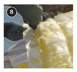
Ensure clean surface for adhesion at overlap seam.
