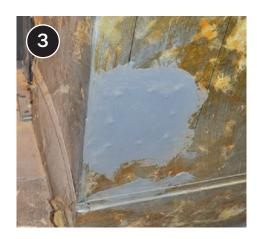
Patch holes in ducts and plenum with appropriate materials (see 19-1 Seal Ducts With Mastic).
