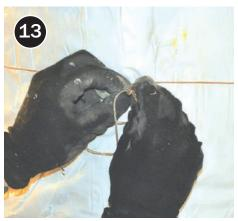
Support insulation to prevent movement over time, securing in place without puncturing vapor retarder.
