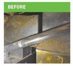
Uninsulated supply and return plenums located in unconditioned spaces allow for energy loss and contribute to occupant comfort issues.
