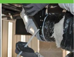
Verify ducts are connected, supported, and air sealed properly.
