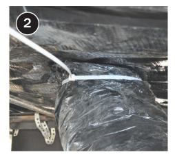
Secure the insulation in place, then seal around the boot to plenum connection with mastic to ensure a complete vapor retarder seal.
