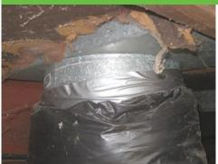
Exposed duct boots are a prime location for energy loss when ductwork is located in an unconditioned space.
