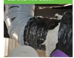
Verify ducts are connected and air sealed at metal connections and any other holes within the liner. When new flex duct is needed, select insulation (duct wrap or flex duct) with a minimum R-8.
