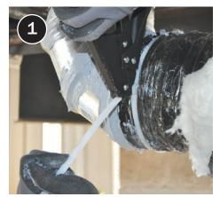
Secure flex duct liner to hard connections with zip tie and tensioner tool. If using duct wrap, follow the same procedure after adding insulation where missing, being careful not to compress the insulation.
