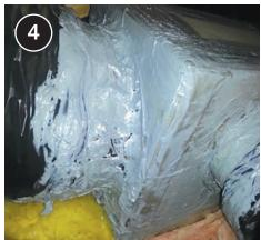
Seal new joints where duct insulation meets plenum using UL-listed material.
