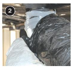
Pull insulation over hard connections as needed.
