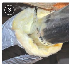
Ensure insulation is not compressed.
