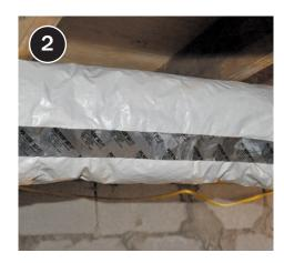
Tape joints to secure insulation in place.
