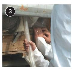
Fill cavity with blown fiberglass insulation, carefully maneuver the fill tube past the belt rail and around electrical boxing/ wiring.
