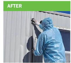
When properly insulated, siding should not bulge or be dented as a result of the installation. Document the location of any pre-existing dents and point them out to the building owner prior to starting a project.
