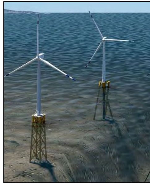
Figure 8: Jacket Foundations, Twisted Jacket on Right [20]
