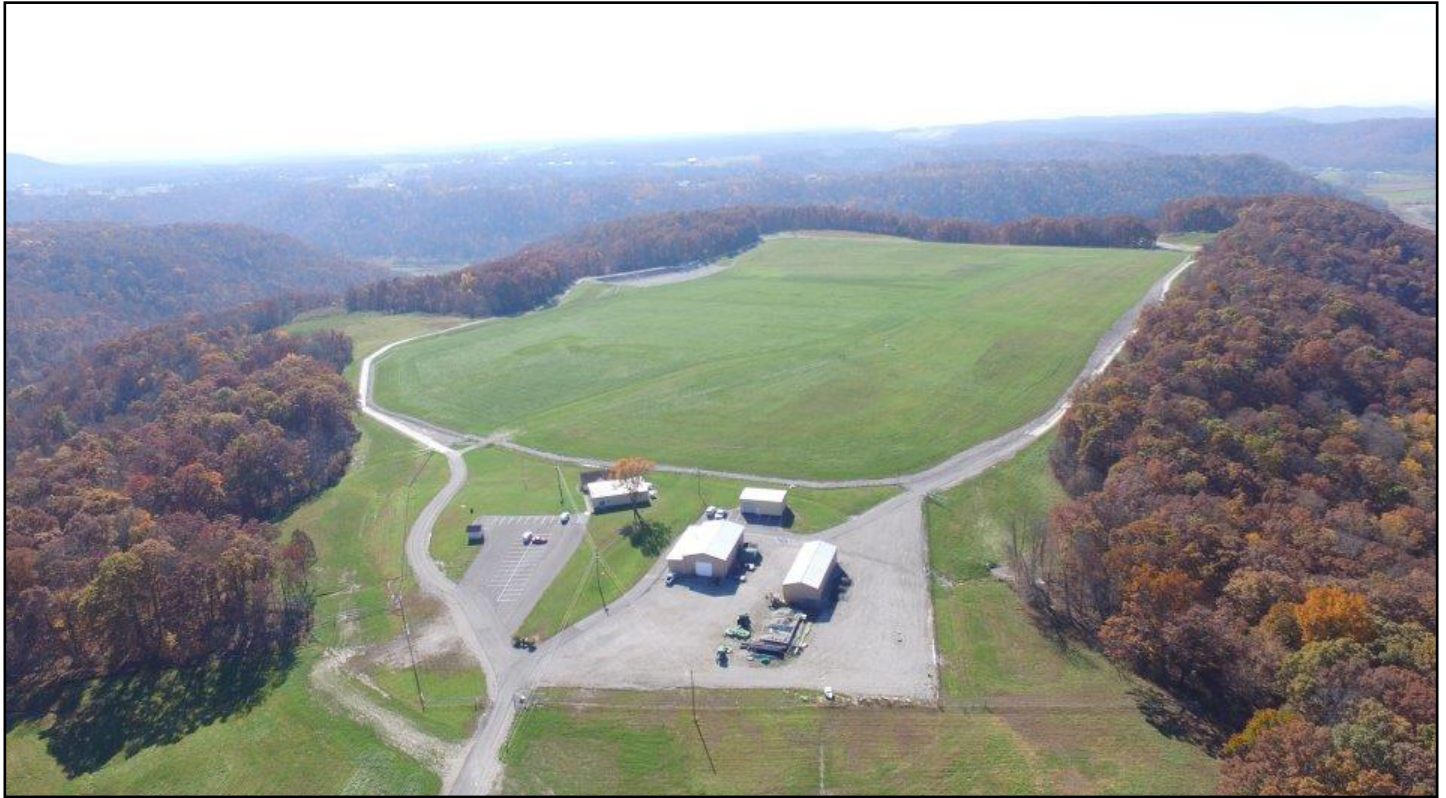
2017 Aerial View of the Maxey Flats Disposal Site; Substantial Completion of the Final Cap Was Achieved in November 2016.
