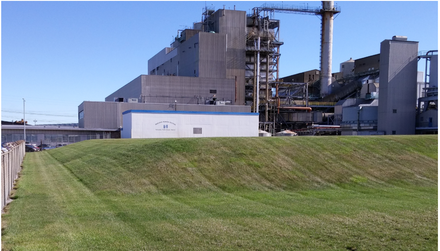
White Building is the Intermediate Heat Exchanger Building. Grassy Area Covers the Belowground Portion of the Decommissioned Reactor Facility.
