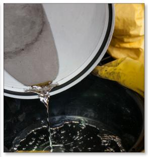
During an EM cleanup project, crews drained, retrieved mercury, and deactivated 8,500 feet of piping of the East COLEX equipment at the Alpha-4 facility at Y-12.
