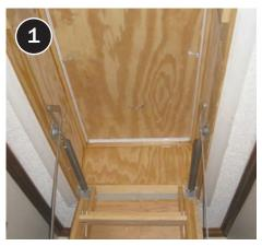
Build cover above and around pull-down stair, taller than final insulation height.
