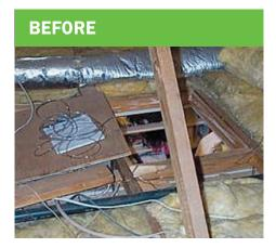
Uninsulated and unsealed attic access points allow conditioned air to escape the home in all seasons and reduce the overall R-value of the attic.
