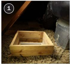
Rigid, durable damming is installed and mechanically fastened in place.
