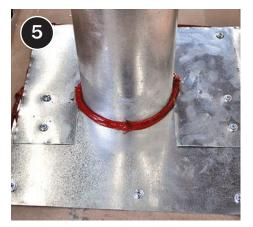
Set the second layer of sheet metal in place. Mechanically fasten the second piece of sheet metal to the first piece using 1/4" sheet metal screws, then secure the metal to the adjacent framing using longer screws.
