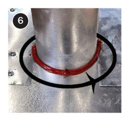
Run bead of high-temperature caulk around the chimney and seal the edge of any remaining gaps to ensure an airtight seal.
