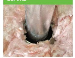
Clear insulation away from chimney or flue.
