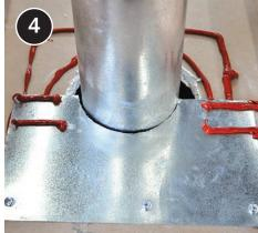
Set the first layer of sheet metal in place, leaving no more that a 1/4" gap around the chimney. Mechanically fasten the sheet metal to the adjacent framing and apply additional caulk where the second piece of sheet metal will overlap.
