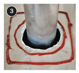
Install a second layer of caulk around the first.
