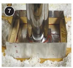
Install a durable fixed dam, at least 2 inches higher than final insulation level, keeping all combustible materials at least 3 inches away from flue or chimney.
