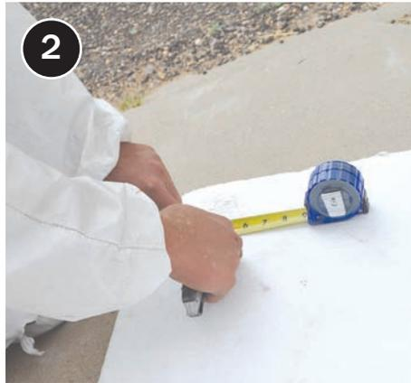
2 Cut material to fit, paying attention to locations of wires and pipes.
