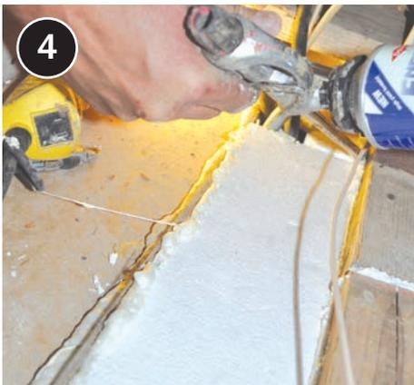
4 Seal all edges with caulk, spray foam, or mastic.
