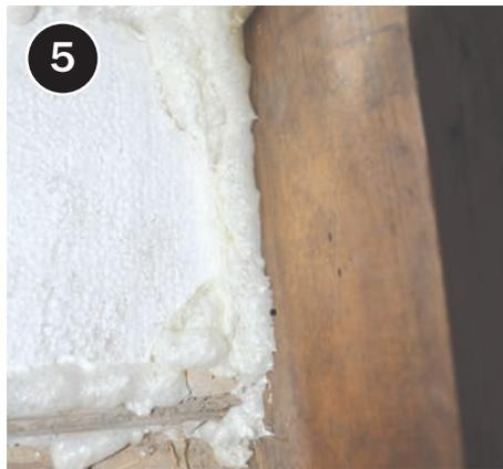
5 Extend sealing to adjacent materials to ensure a complete air seal.
