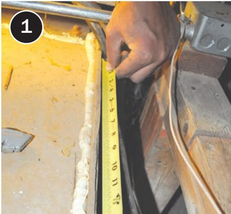
1 Measure the opening of the chase in a location that will maintain the pressure plane.
