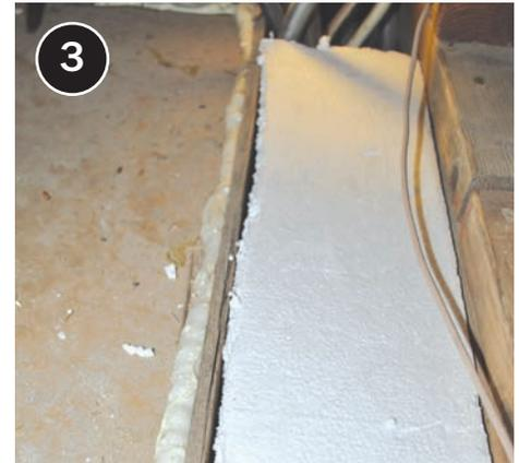
3 Friction fit the piece and mechanically fasten where feasible.
