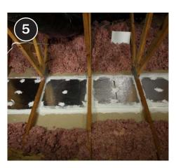
The pressure boundary is now aligned and ready for insulation.
