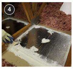
Seal seams, edges, and the tops of all mechanical fasteners.
