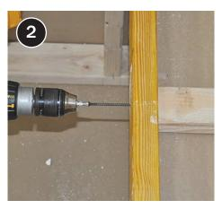
If necessary, attach bracing across joists securely, spacing no more than 24 inches apart.
