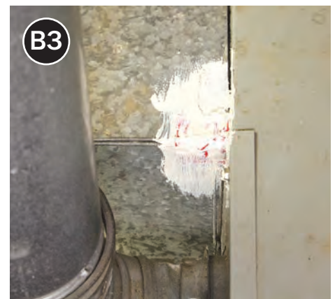
Apply mastic over the tape.
