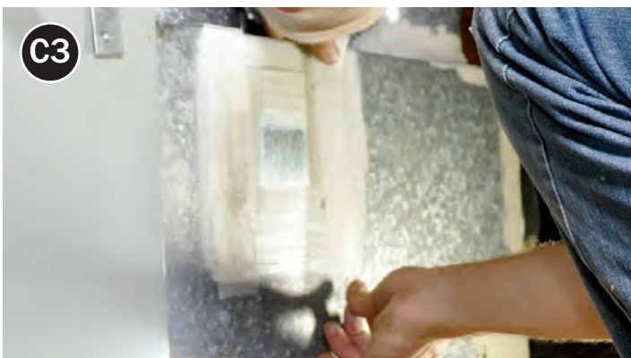
Apply mastic over edges and fasteners of patch and push fiberglass mesh into it.
