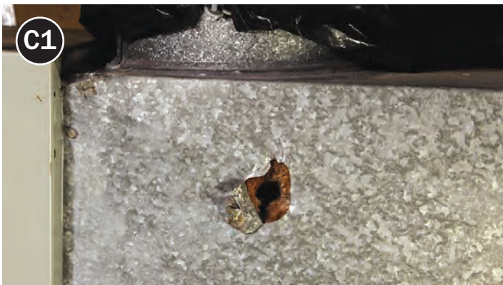
Larger holes require a different process.
