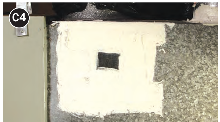
Apply additional mastic over mesh, extending at least 1 inch past tape and seam in all directions.
