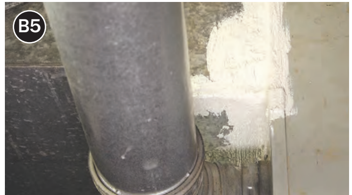
Apply additional mastic over mesh and tape, extending at least 1 inch past edges of tape in all directions.
