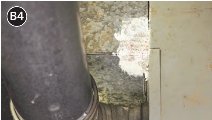
Push fiberglass mesh into the mastic.
