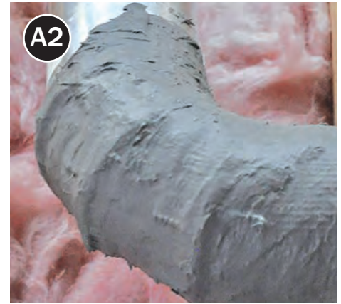
Apply mastic over all mesh tape and all gaps, seams, joints, etc.
