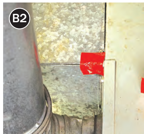
Apply temporary UL-listed or mesh tape as a backer to hold mastic.
