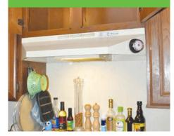
Kitchens and bathrooms must be ventilated to control moisture, vapor, and combustion gases.
