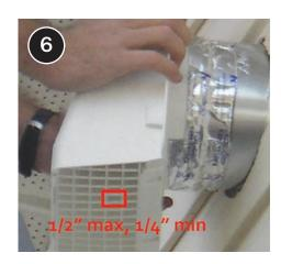
Chose appropriate exterior termination to match size of duct while minimizing water and pest intrusion. Seal around exterior termination as needed.
