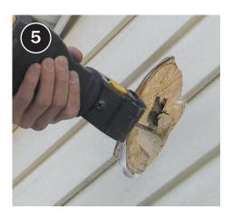
Locate exterior vent based on duct run and size hole less than ½ inch larger than duct.
