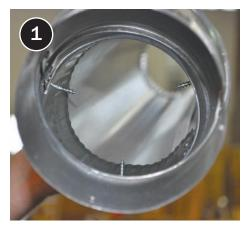
Fasten rigid duct using three equally spaced screws. Ducting should be 28-gauge or thicker.
