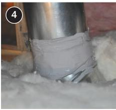
Cover mesh with a layer of mastic to seal all joints.
