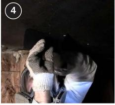
Cut access holes to ensure entire cavity will receive continuous and consistent insulation.
