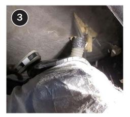
Based on installer preference and site conditions, bellies can be insulated from underneath or the edge when using a fill tube or pipe.
