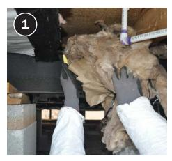
Remove old insulation if necessary and make repairs as needed in preparation for belly patch material.
