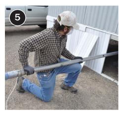
Fill entire belly cavity to prescribed R-value while ensuring plumbing has sufficient insulation value to prevent condensation or freezing.
