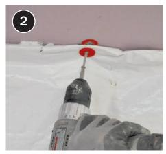
Mechanically fasten belly repair material. Seal all seams and edges.
