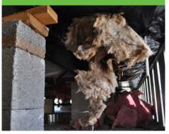
Determine if belly repairs are needed and make sure no plumbing or other issues preventing additional insulation exist. All duct sealing should be complete and the direction of the floor joists (crosswise or lengthwise) must be identified.
