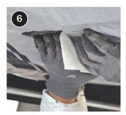
Apply waterproof, permanent adhesive to patch for belly wrap, with patch sized at least 3 inches larger than hole in barrier.
